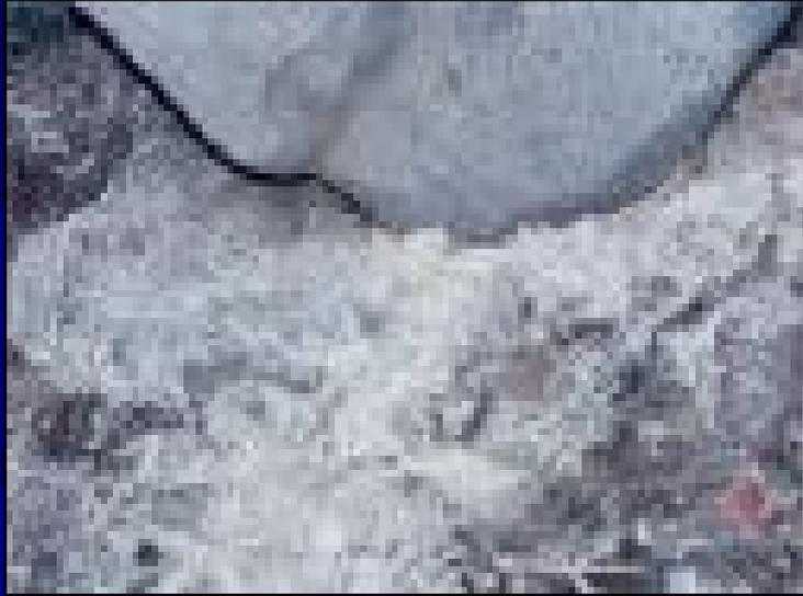
**Salt crystallization under the stone surfaces**
