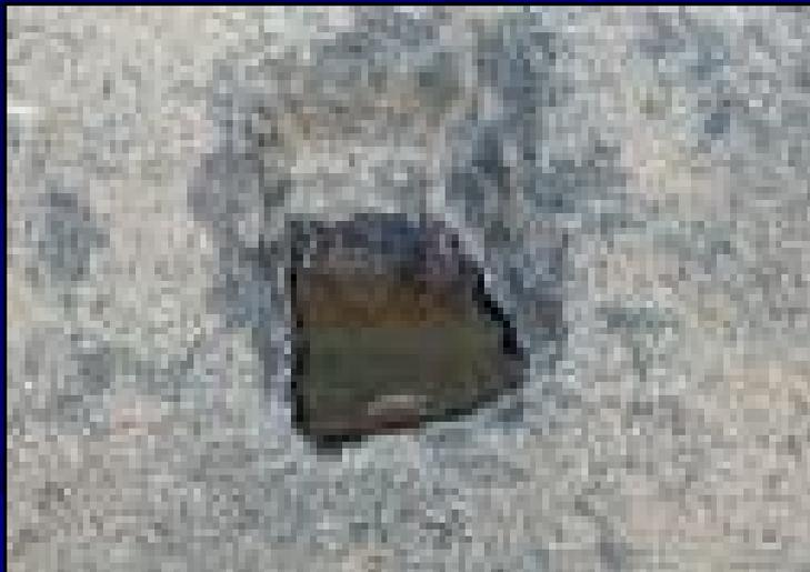
**Frost action resulted from freezing of water sources**
